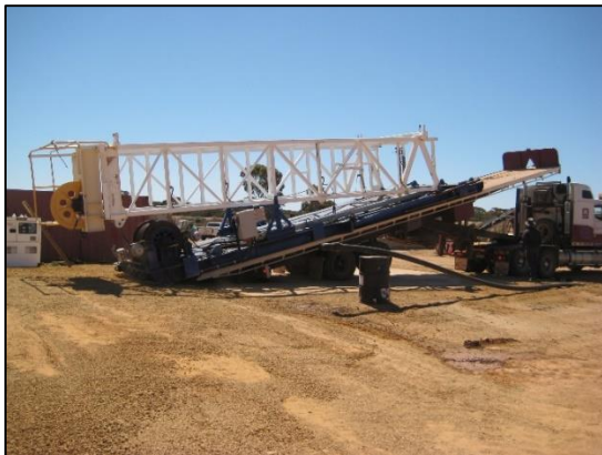
Unloading headframe at the Radio shaft collar
